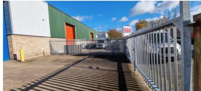
Rear external area
