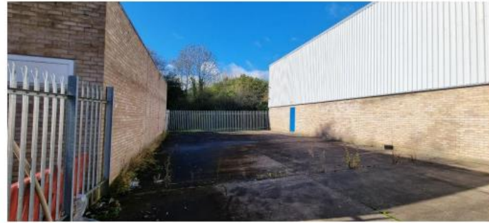
Rear external area
